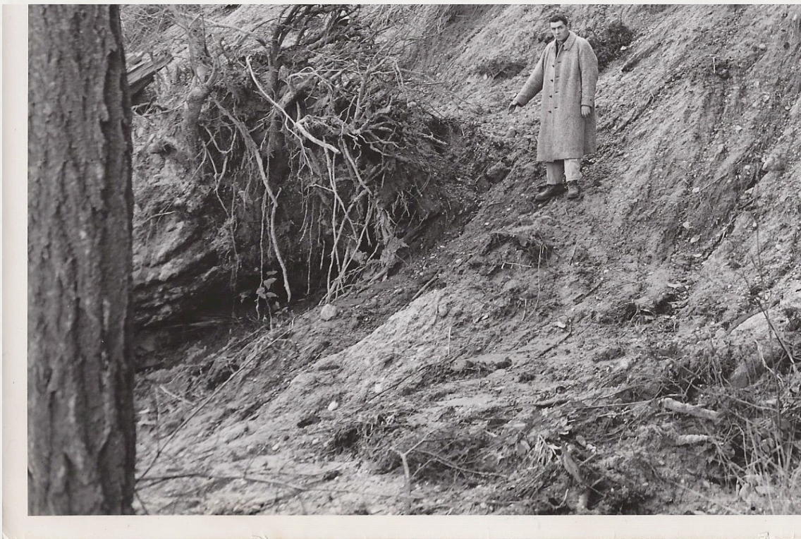
Don MacDonald checking out slide damage.
